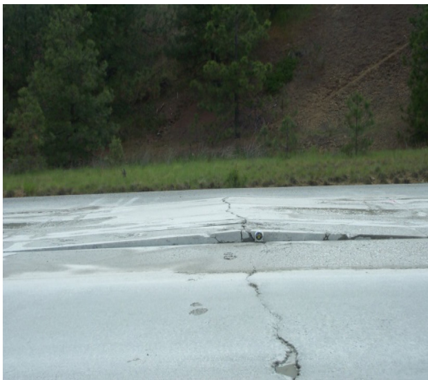
Figure 2.12: An illustration of blowup in JPCP (Harrington et al., 2018).
