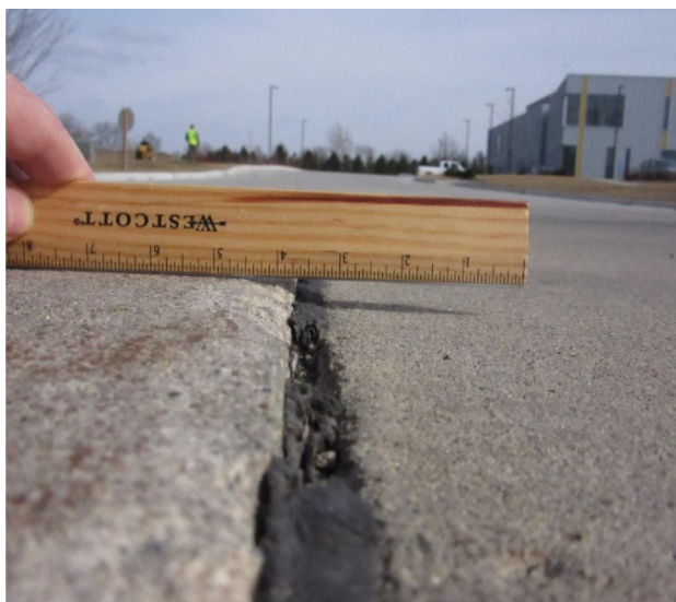
Figure 2.10: Faulting in JPCP (National Concrete Pavement Technology Center (used with permission)).
