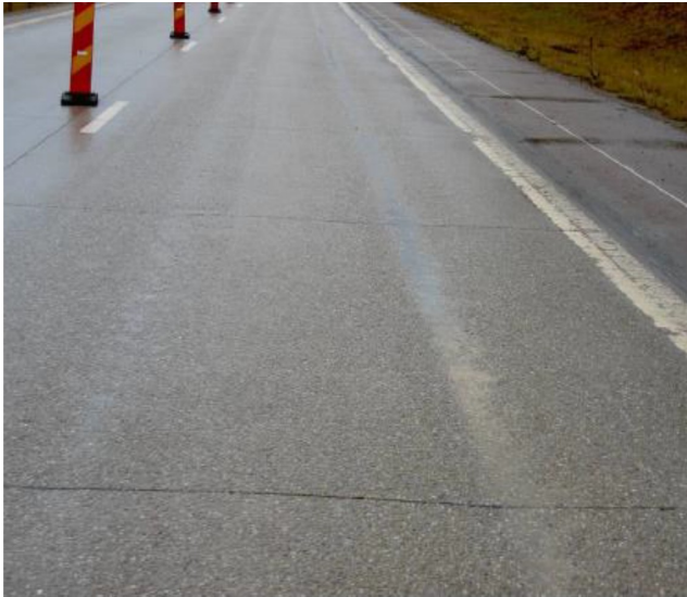
Figure 2.13: Rutting due to studded tires in JPCP used with permission of Ellen Dolk (Hultqvist and Dolk, 2014).
